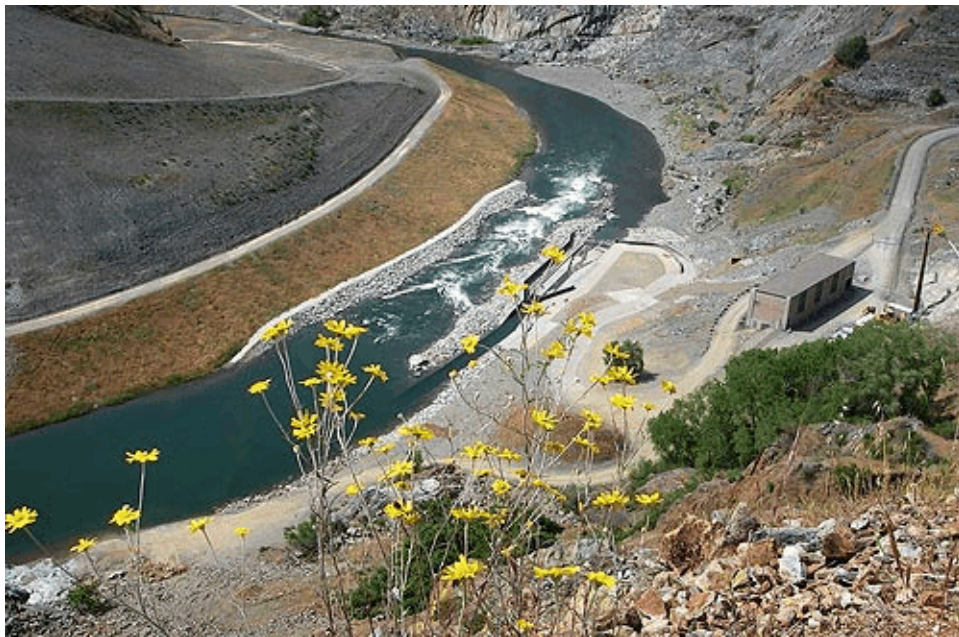
The Auburn Dam may never be built at this site on the American River, 35 miles northeast of Sacramento. Construction has been a local issue since Congress authorized it in 1965. Auburn Journal
